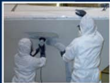
Custom fiberglass and gelcoat repairs.
